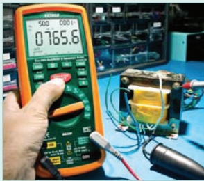
Measure the insulation resistance of transformer windings
